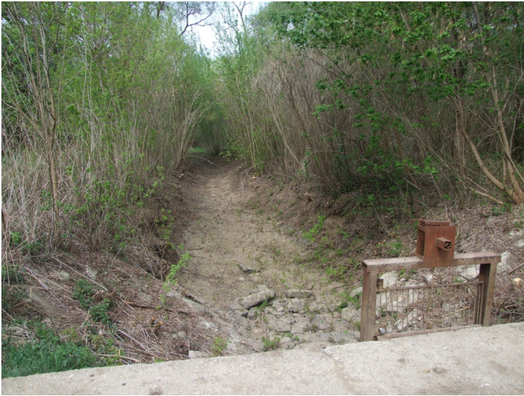
Fig. 13. The dried-out canal between the Marót-zugi-Holt-Tisza and the Mocsolya in the spring of 2019 (Photo: György Dévai, April 20, 2019)
