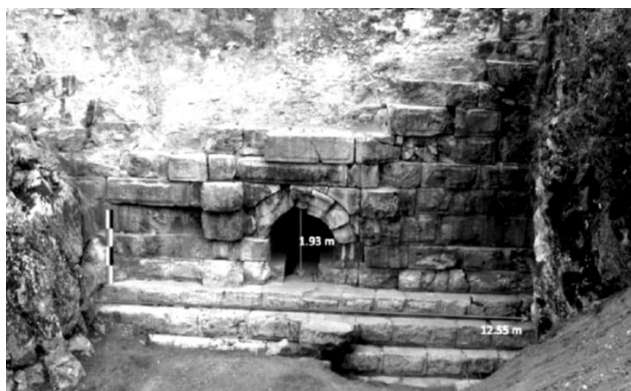
Fig. 3. The Örükaya Dam after the excavations (after İPEK, SÖKMEN 2018, 234).
