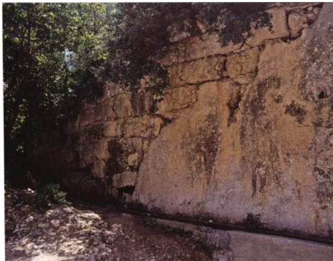
Fig. 7. The Seleucia Dam (after TORUN 2020, 150, fig. 61).
