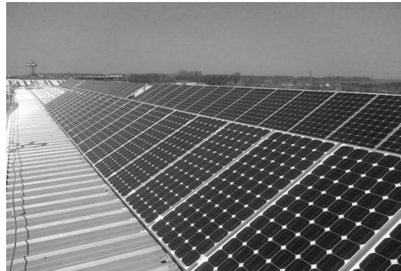
Figure 1: The installed PV cells
