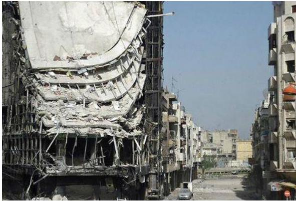
Figure.2 – Destruction in Homs, Source: Shaam News Network
