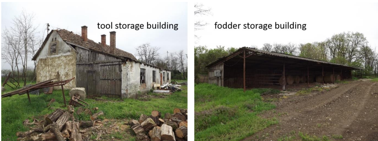
a tool storage building to be demolished, number 07
