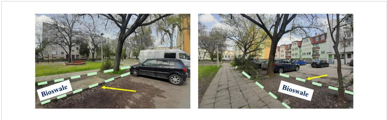
Figure 20. Redirection of Runoff Toward Playground for Bioswale Integration
