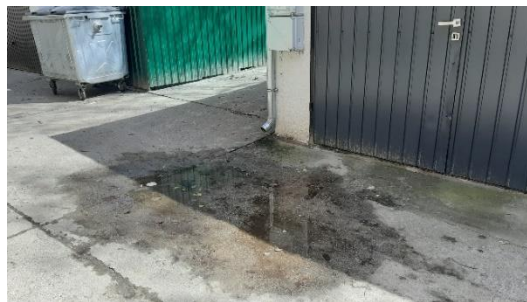
Figure 8. Puddle formation due to roof drainage discharge onto the asphalt surface
