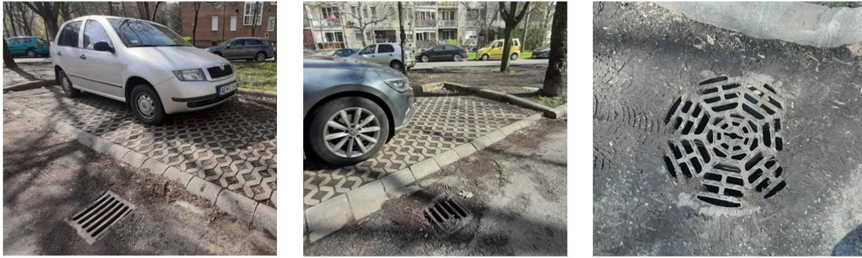
Sediment accumulation around catch basins indicates limited retention capacity and prolonged runoff time during heavy rainfall. Additionally, excess water from the saturated pervious layer may contribute to overflow.
