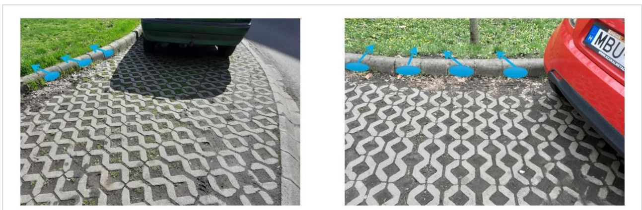
Figure 16. Curb cuts applied to channel runoff into a rain garden
