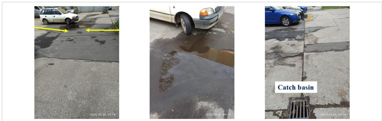
Figure 15. Water Accumulation and Deteriorated Concrete in Parking Lot 4
