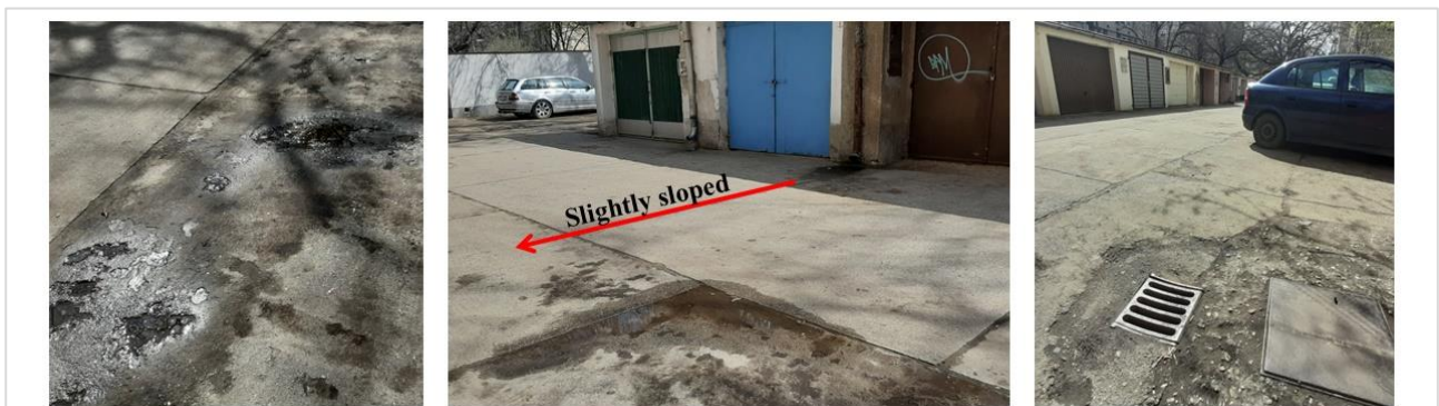
Figure 9. Water accumulation due to deteriorated concrete sections
