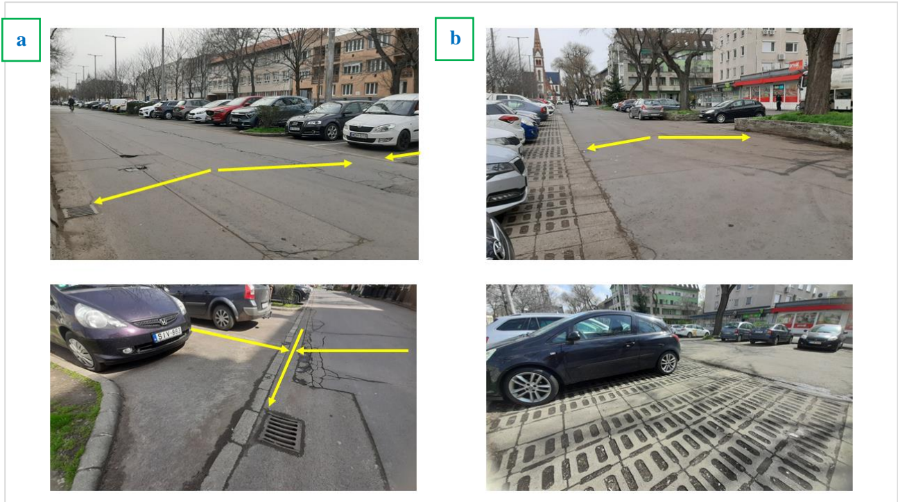
Figure 12. Section of the parking lot with a) sloped concrete and b) interlocking pavers
