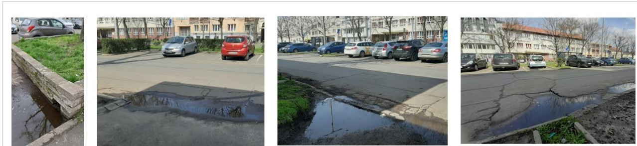
Figure 13. Water accumulation after rainfall along parking lot 3
